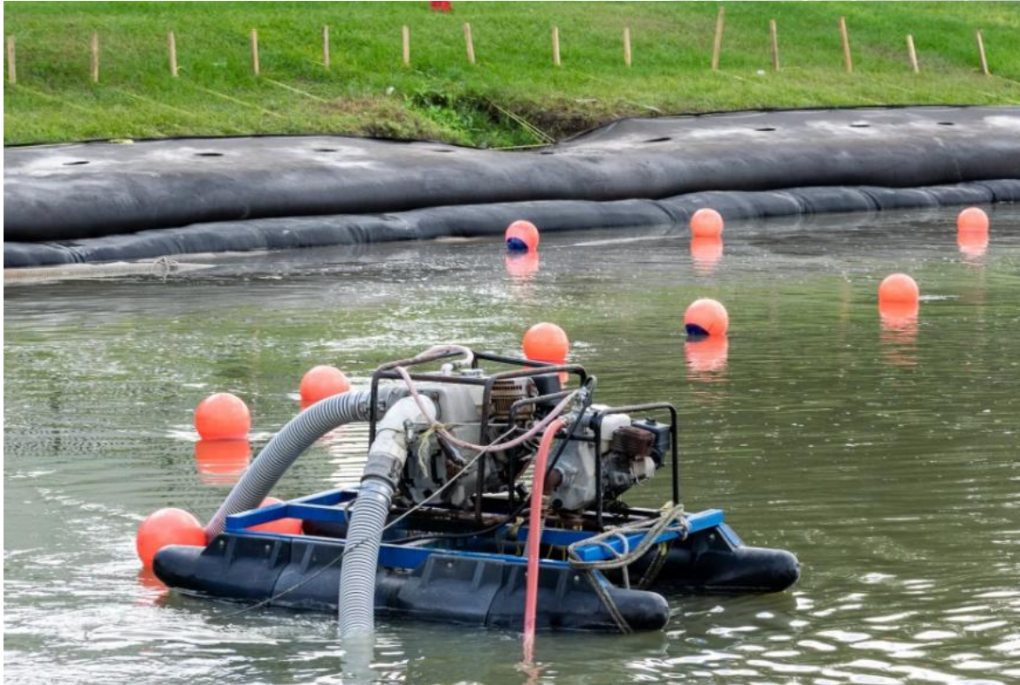
Dredging Machine and Geotube Stacking
