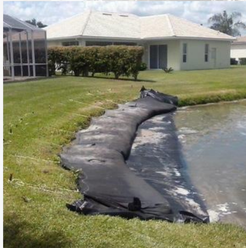
Filling GeoSOX with Sediment
