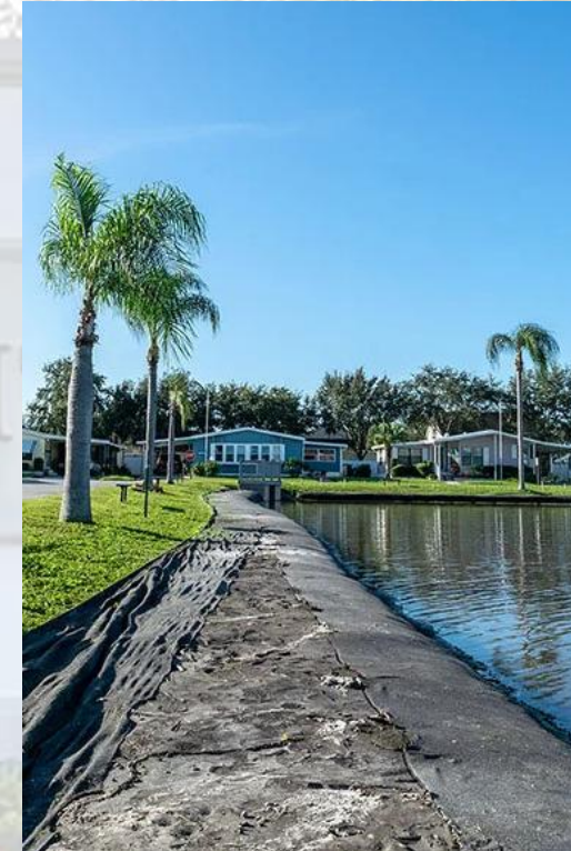
Geotube Split for Grading
