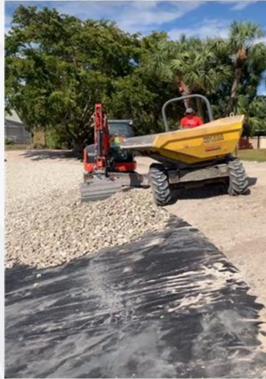
Stone Being Placed on Lake Bank
