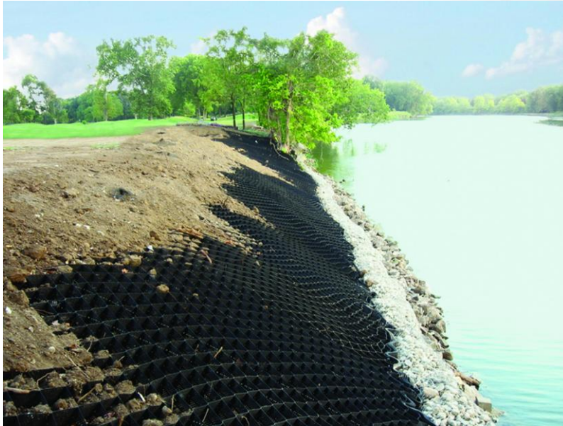
Geoweb Infill Installation
