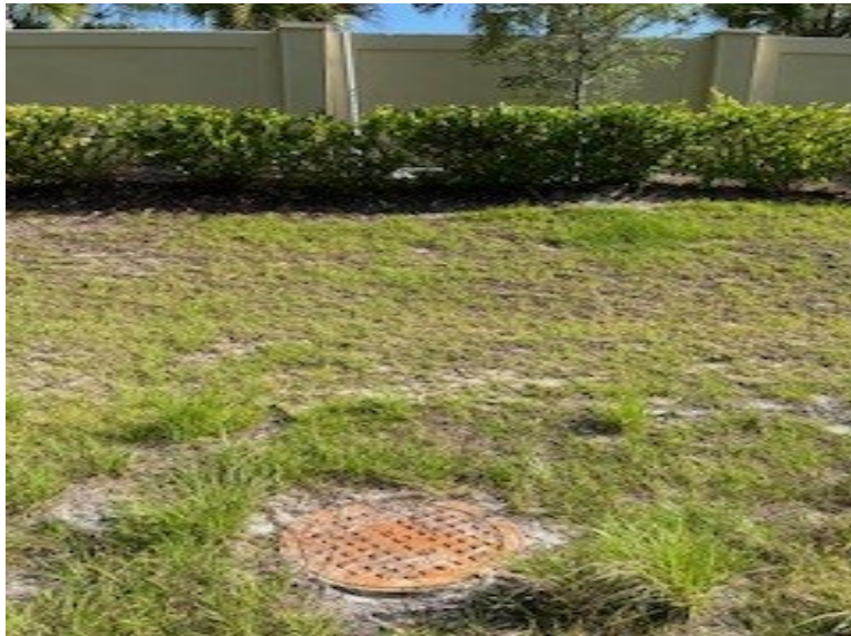
JUNCTION MANHOLE ON SOUTH SIDE OF WALL
