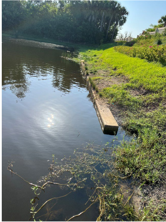
HEADWALL IN LAKE #55
